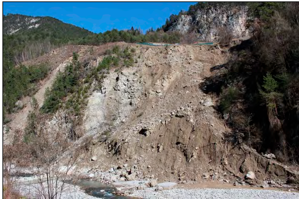
Figure 10. Frontal view of the landslide showing the complex composition of the soil involved.
