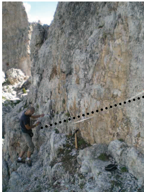
Fig. E.2. Approximate position of the horizontal scanline at the basement of the western side of the Torre Latina pinnacle: Site 2. The trace of the scanline is drawn-in by hand. The horizontal scanline survey was carried out from left to right over 5.00 meters.
