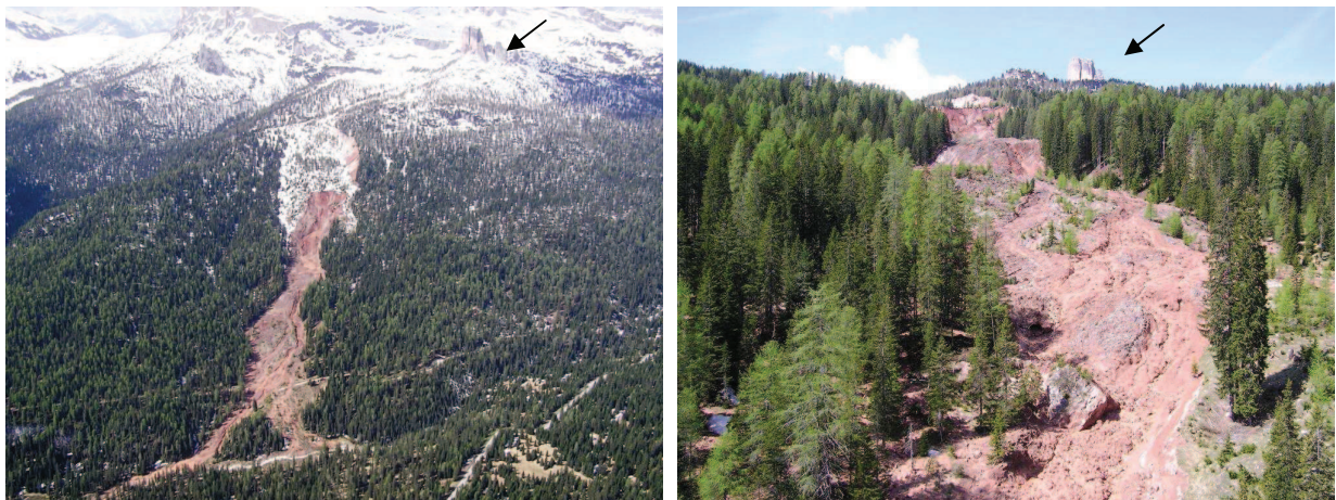
Fig. 2.6. Pictures of the reactivated mudflow which broke off on May 2009 during snow melting period. The mudflow is located about 1400 m from the Cinque Torri group, indicated on pictures (image courtesy of C. Baglioni).
