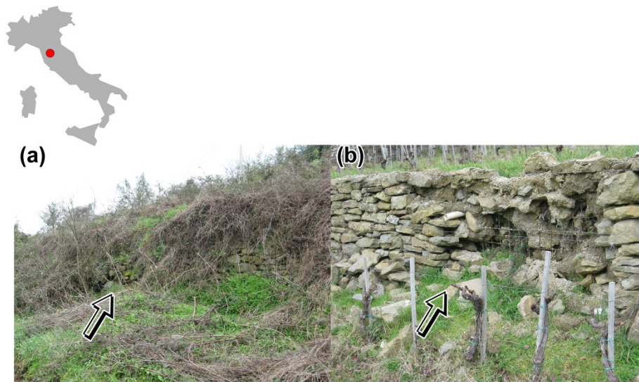
Fig. 16. Examples of terrace abandonment (a) and lack of maintenance of terraces with consequent failure (b), of a vineyard located in the Tuscany region (central Italy) (photo by S. Calligaro).
