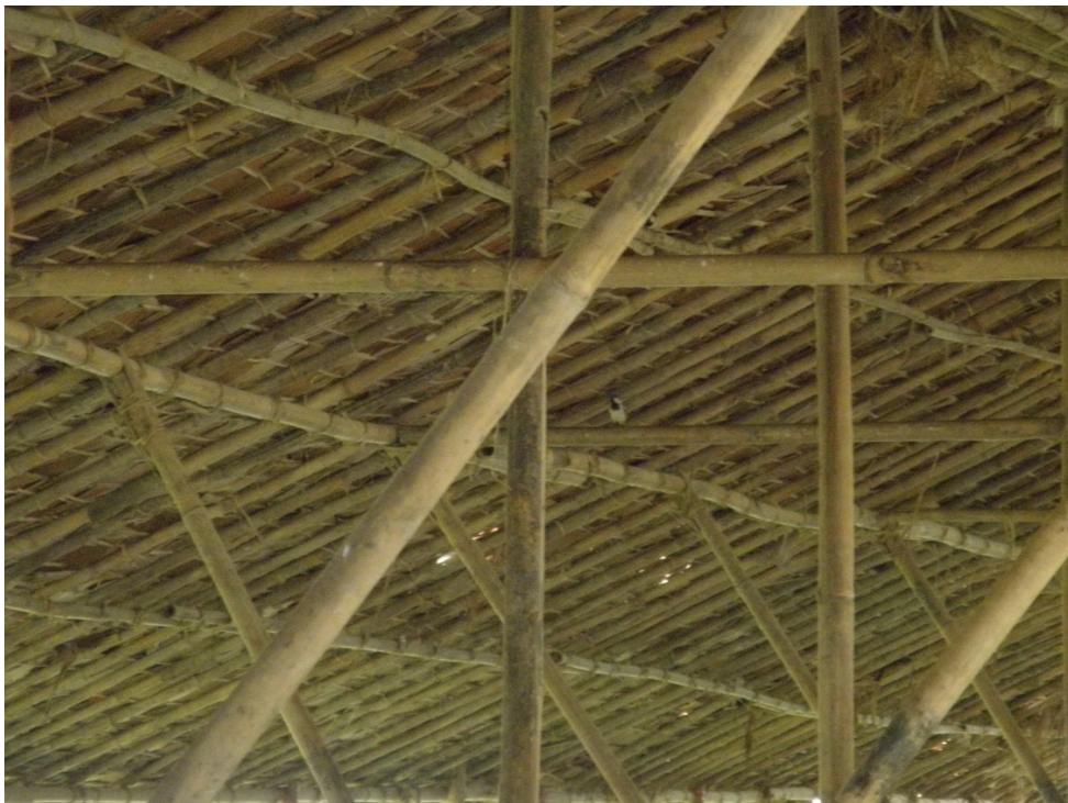
Figure 5: Roof made of palm leaves on a bamboo frame.
