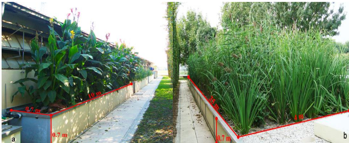
Figure 2.2a - General view of VF unit and cell details Figure 2.2b - General view of HF unit and cell details, August 2010.
