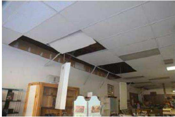
Fig. 7 a): Damage reported from L'Aquila earthquake in 2009 (Magliulo, 2009); b): Damage reported after New Zealand earthquakes in 2010 and 2011 (Dhakal et al., 2013); c) and d): Damage reported from the 22nd February 2011 Christchurch earthquake (Dhakal et al., 2011); e): Damage reported after Napa (CA) earthquake in 2014 (Gilani et al., 2015); f): Damage reported after the 2010 Baja earthquake (Gilani and Takhirov, 2011).
