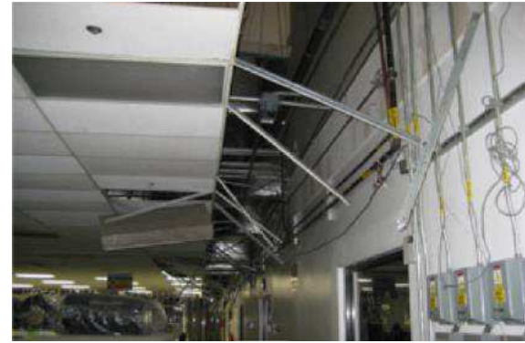
Fig. 7 a): Damage reported from L'Aquila earthquake in 2009 (Magliulo, 2009); b): Damage reported after New Zealand earthquakes in 2010 and 2011 (Dhakal et al., 2013); c) and d): Damage reported from the 22nd February 2011 Christchurch earthquake (Dhakal et al., 2011); e): Damage reported after Napa (CA) earthquake in 2014 (Gilani et al., 2015); f): Damage reported after the 2010 Baja earthquake (Gilani and Takhirov, 2011).
