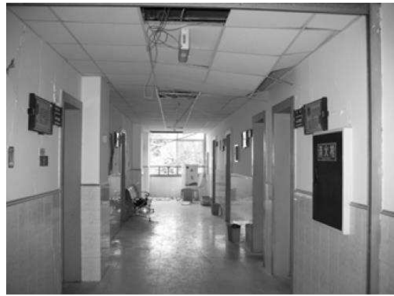
Fig. 10 a): Interaction between bulkheads and ceiling after New Zealand earthquakes in 2010-2011 (Dhakal et al., 2013); b) Damage reported after L'Aquila earthquake in 2009. (Magliulo, 2009); c) Ceiling panel dislodged in the Olive View Medical center, Sylmar, California, photo by Robert Reitherman. (Taghavi and Miranda, 2003); d) Damage reported after the Sichuan Earthquake, China, in 2008. (Glasgow et al., 2010)
