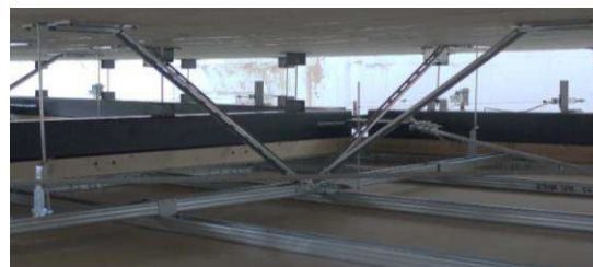
Fig. 46: Plast Doub system: a) placement of the runners and the plasterboards and details of the bracket and the hanger rods, b) picture of the installation of primary and secondary runners, c) installation of the seismic bracing system, d) picture of a specimen.
