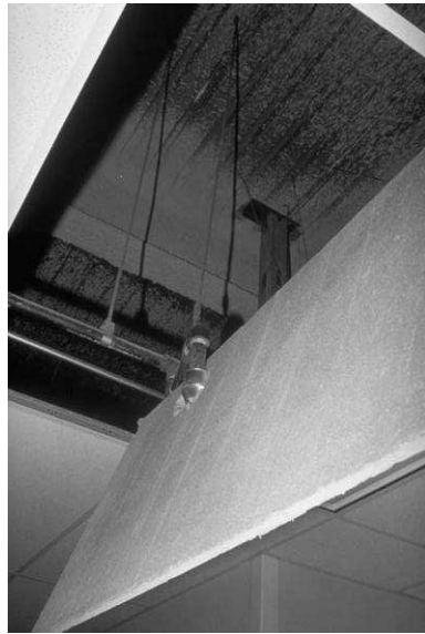
Fig. 10 a): Interaction between bulkheads and ceiling after New Zealand earthquakes in 2010-2011 (Dhakal et al., 2013); b) Damage reported after L'Aquila earthquake in 2009. (Magliulo, 2009); c) Ceiling panel dislodged in the Olive View Medical center, Sylmar, California, photo by Robert Reitherman. (Taghavi and Miranda, 2003); d) Damage reported after the Sichuan Earthquake, China, in 2008. (Glasgow et al., 2010)
