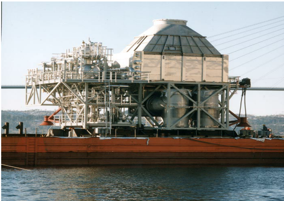
Figure 2.8: The double-inlet, single lift Oseberg WHRU-SG [85].
