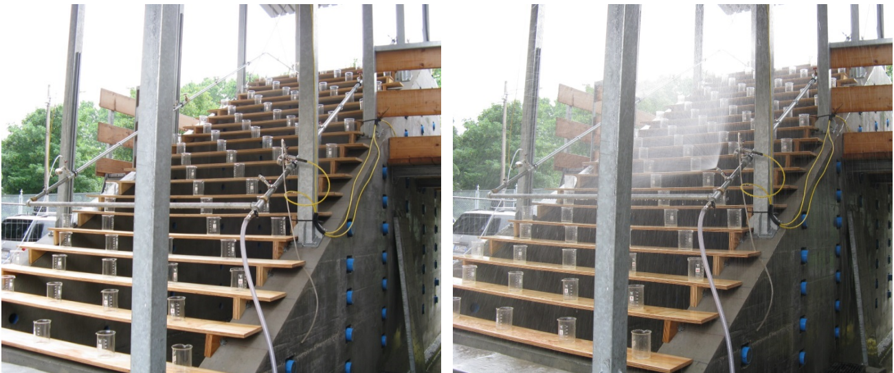
Figure 2-14. An image of the (on the left) rainfall simulator installed on the artificial hillslope, and (on the right) during an experimental test for measuring the rain intensity.
