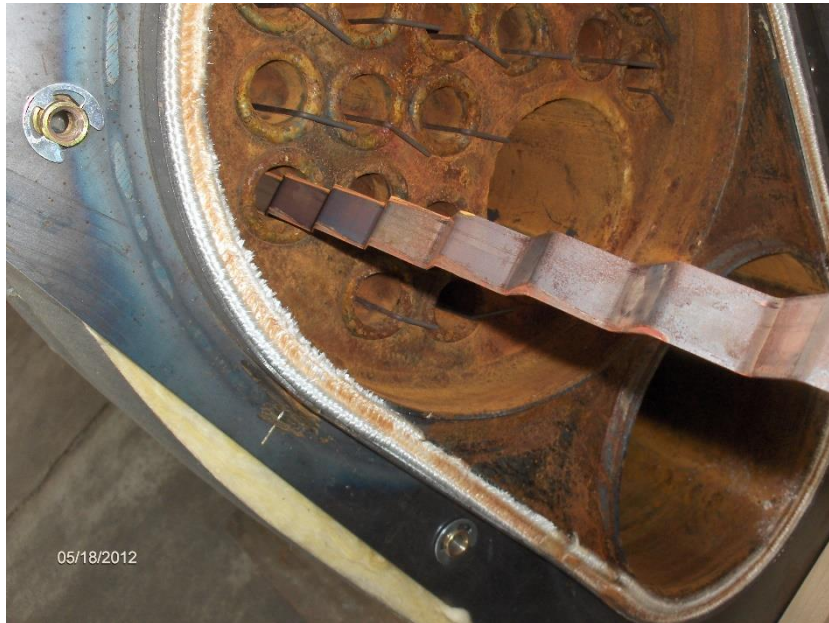
Figure 1.2.2.1. Photo of the wave turbulators.
