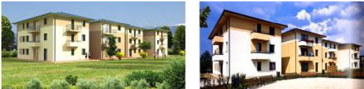
Figure 16-1. Views of the considered three-story building
