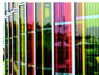
Fig. 1.2.3 Windows of the conference center EPFL (École polytechnique fédérale de Lausanne) in Switzerland with colorful embedded organic DSSC.
