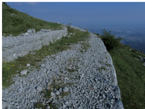
Figure 2. Present condition of a well preserved military road
