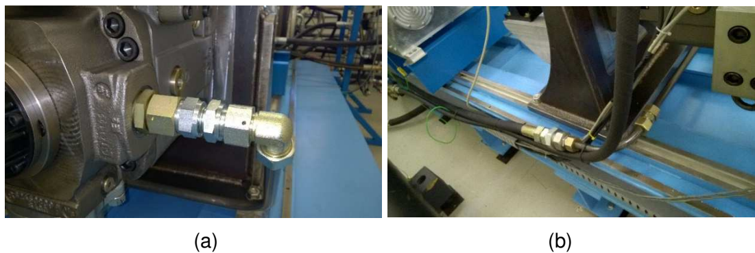
Figure 6.13: Check valves in the same low-pressure line.
