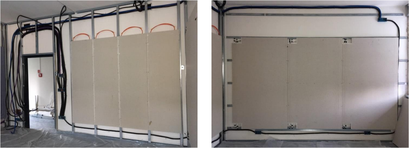
Figure 6.11 - Construction phase of the radiant dry walls.
