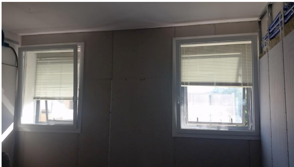
Figure 6.14 - The external wall after the installation of the new windows.
