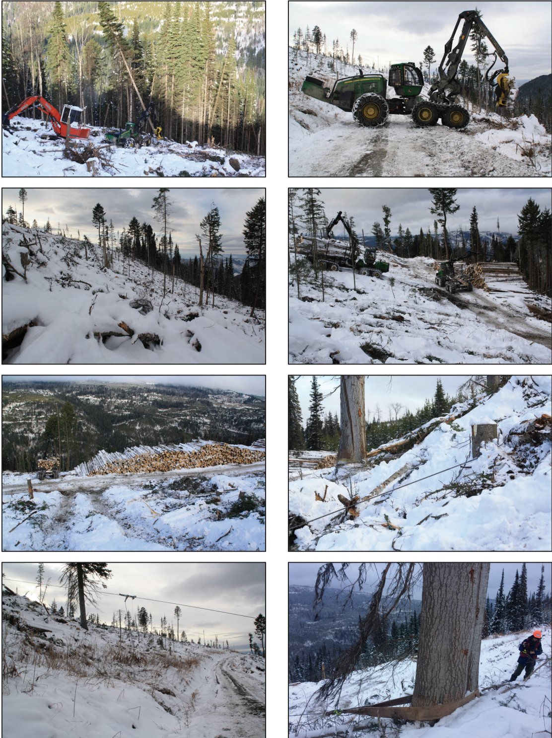
Figure 6.15: Photos of Site O. From the top left: Winch-assist harvesting operations; Harvester; Harvested area; Unloading at the Landing; Winch-assisted forwarder close to the landing; Deviating system used to center the cable on the trail; Cable tensile force monitoring system; Anchor
