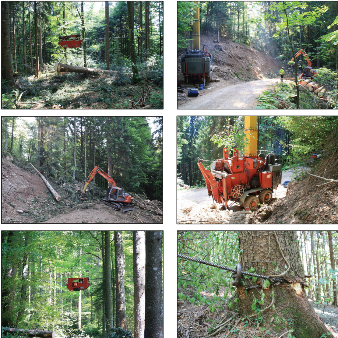
Figure 6.4: Photos of Site D. From the top left: Lateral skid; Landing; Unloading; Cable yarder; Carriage; Anchor
