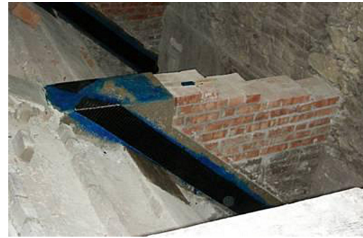
Figure 2.36: Reinforced transversal ribs on the vaults of the Ducal Palace in Urbino (Modena et al. 2009)
