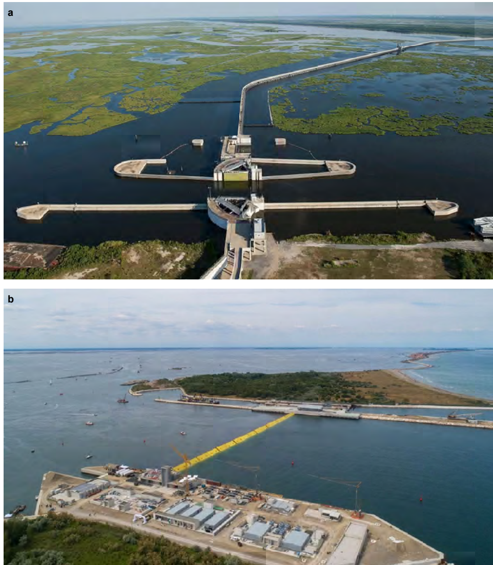
Figure 1.8: Examples of storm-surge barriers. a, Inner Harbor Navigation Canal (IHNC) Lake Borgne Surge Barrier designed to protect New Orleans, Louisiana, US. Photo: engineering-channel.com . b, Barrier of the Mo.S.E. system at the Chioggia inlet, Venice Lagoon, Italy. Photo: mosevenezia.eu
