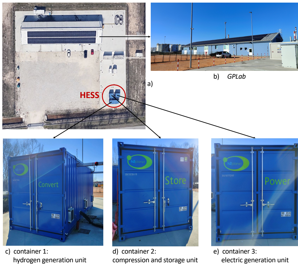
Fig. 2 – GPLab and HESS: a) a satellite view of the laboratory (source: Google Maps); b) laboratory building; c) Convert: hydrogen generation unit (HGU), where hydrogen is generated and purified; d) Store: compression and storage unit (CSU); e) Power: electric generation unit (EGU).
