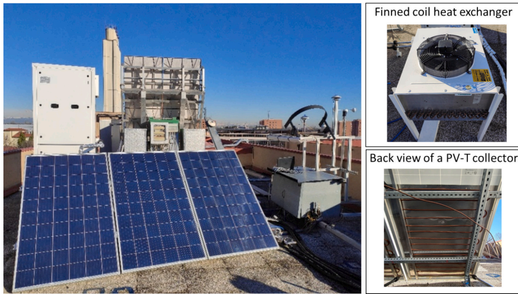
Fig. 1. Pictures of the SA-DSHP prototype with details of the finned coil and of the back view of a PV-T collector.
