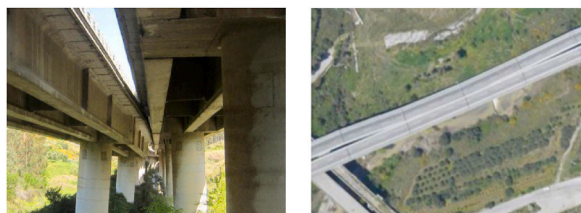
Fig. 1. The Himera viaduct in Sicily [10].
