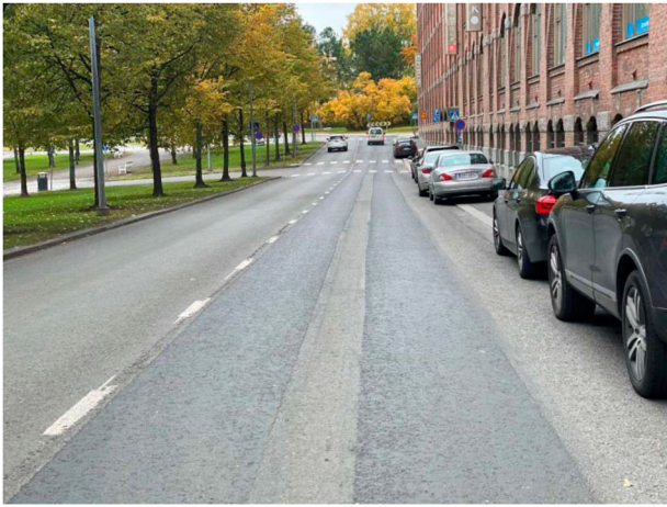
Figure 1. Example of typical results of rut-remix (RUT-REM) treatment (Väylä, 2019).
