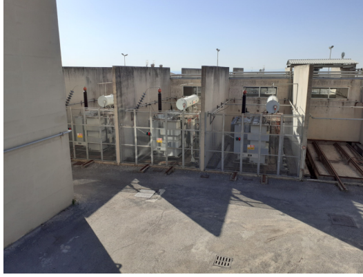
(a) View of building 90 from 📷 labeled “view 1” in Fig. 2.3.
