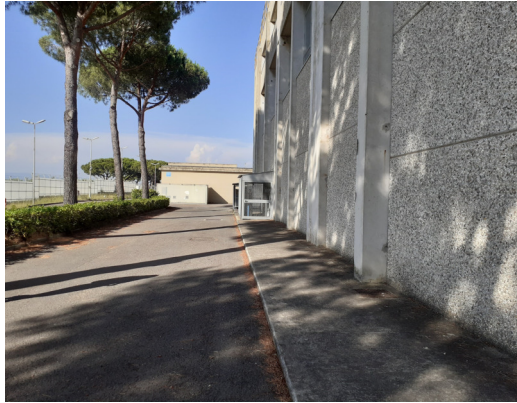
(b) View of building 87 from 📷 labeled “view 2” in Fig. 2.3.
