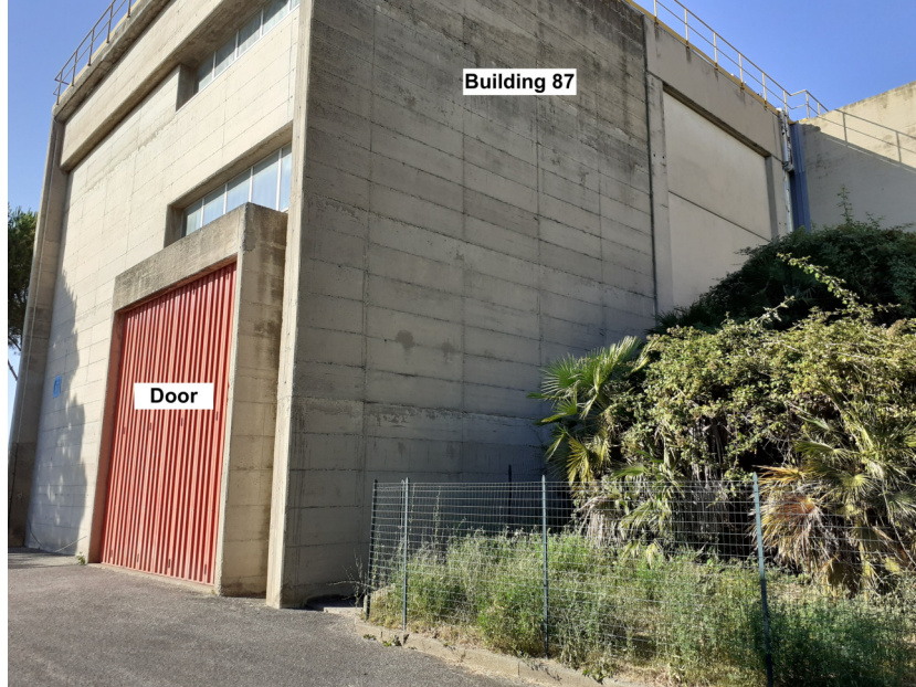
Figure 6.1: Photograph of the west door of building 87 through which the HDV-HVB connection will pass.
