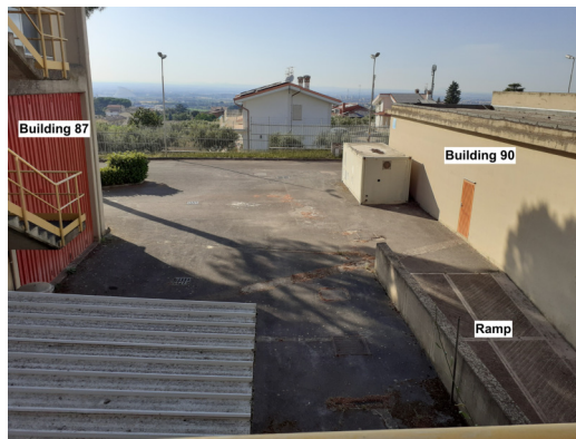
(c) View of ramp between building 87 and building 90 from 📷 labeled “view 3” in Fig. 2.3.
