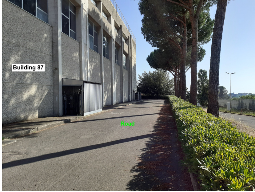
Figure 2.9: Photograph of part of wall of building 87 in which the construction of the rack is planned.
