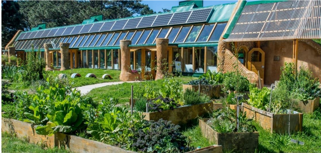
Figure 19. Public School No. 294 (Una Escuela Sustentable, 2021).
