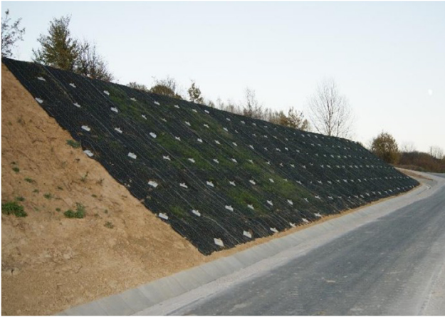
Fig. 1. Example of an anchored mesh facing along a road embankment.
