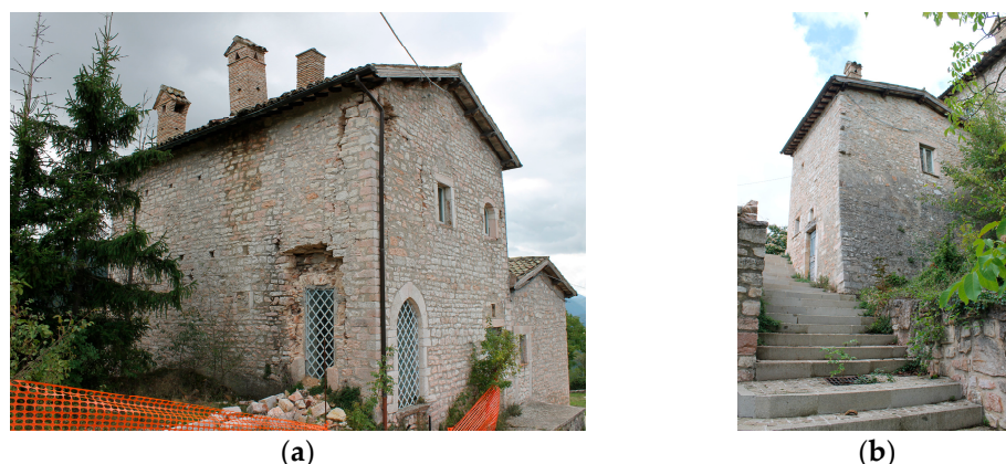
Figure 15. MSB external views: (a) from north-west; (b) from south-east.
