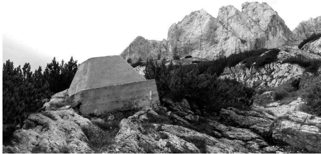
Figure 21.1. Str.obs in the Dolomites. One of the plinths remaining from old chair lifts on the Marmolada slopes Source: Photo by Chiara Quaglia, 2016
