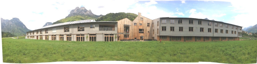
Fig. 17. The school building in Agordo (from south).
