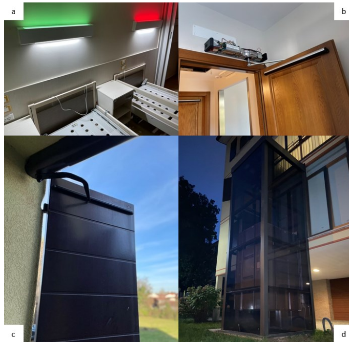
Figure 2.1. Useful elements for the reduction of architectural barriers. Figure 2.1.a shows the controllable electric beds and the lights placed above them; figure 2.1.b shows the motor that allows the automatic opening of doors; Figure 2.1.c shows the window shutter engine; Figure 2.1.d shows the elevator that will take the residents inside the apartment.
