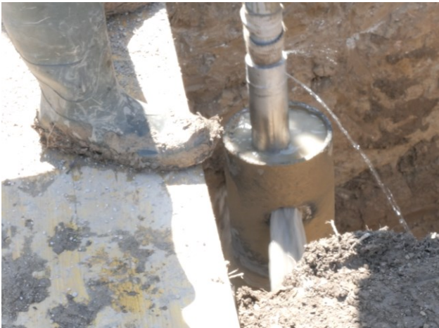
(c) GHE insertion using the excavator and pressurized water.
