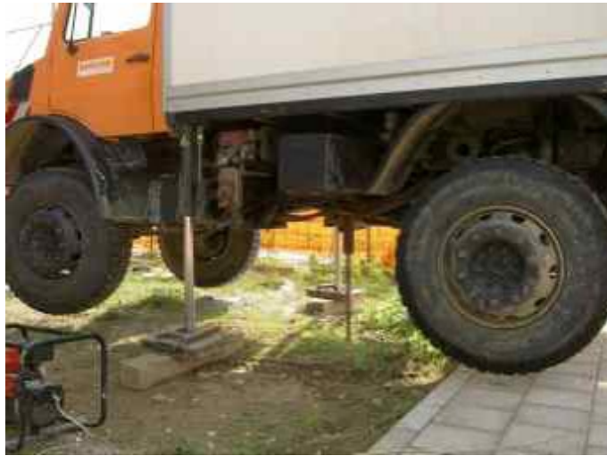
Figure 6: Direct installation of a 50 mm diameter coaxial GHE in SS304-SS304L stainless steel using a penetrometer (methodology patented by Tecnopenta srl – RED srl).
