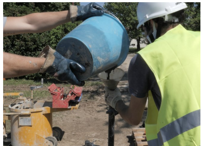
(f) Closing the open end with cement.
