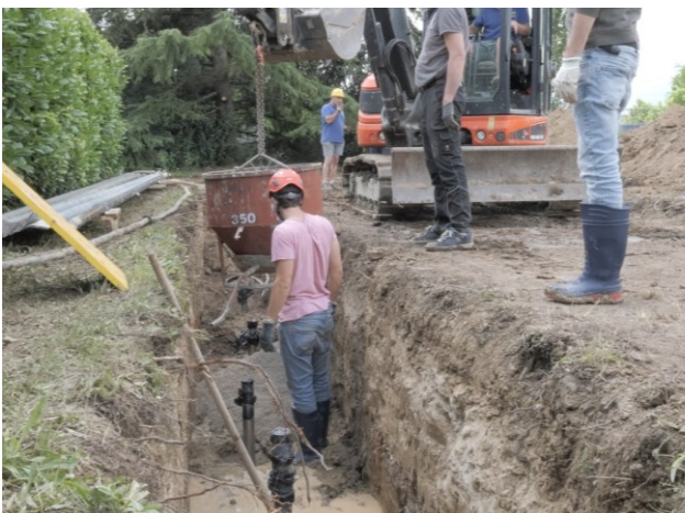
(e) Filling the borehole.
