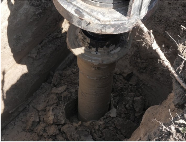
(a) Drilling and casing from -1.50 (pit depth) to -8.50 m below g.l..
