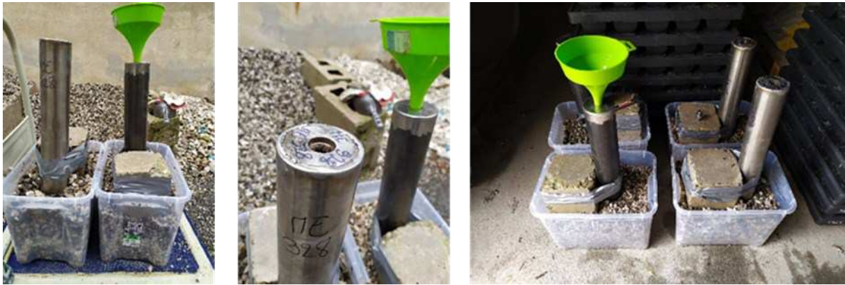
Figure 25: From left to right securing of the well points in gravel and fine gravel, top view of the well point with the space for inserting the grout, preparation for the grout filling.
