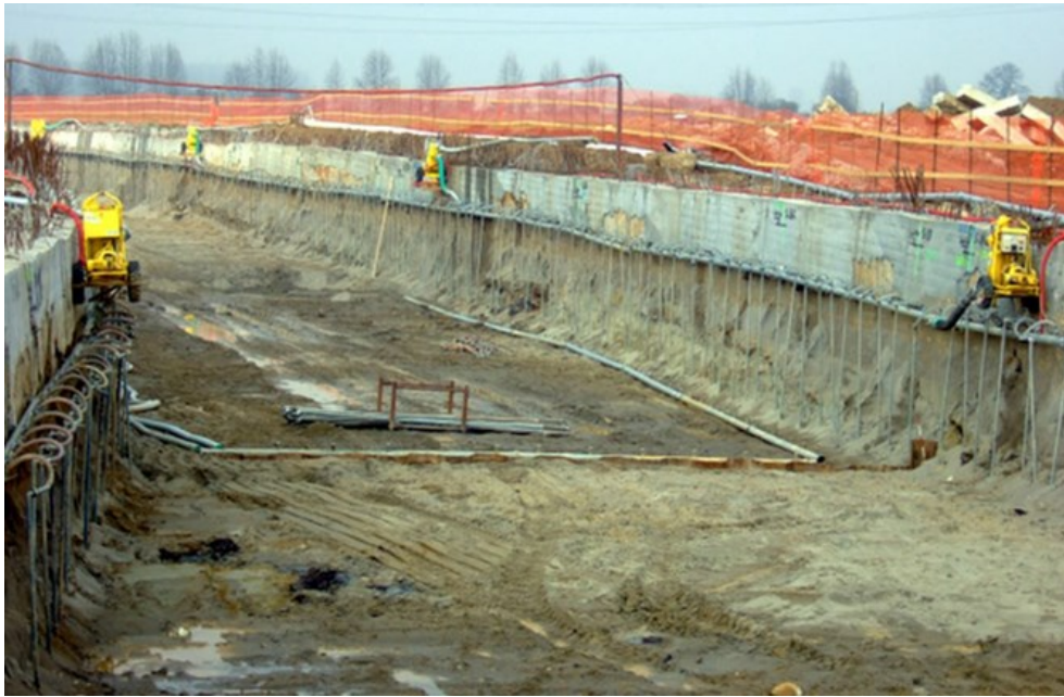
Figure 2: On field well-point system for dewatering applied to a wide excavation
