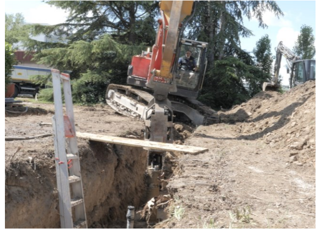
(b) Positioning of the GHE and connection between GHE and hydraulic pump.
