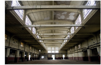
Interior view of the main building
