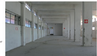
Interior view of the first floor
