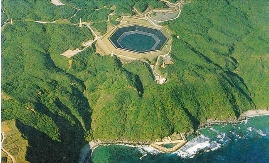
FIGURE 1.5: Bird-eye view of the Okinawa sPSHP. The upper reservoir has an octagonal shape, and tetrapods are placed at the outlet of the tailrace for protection against waves [64].
