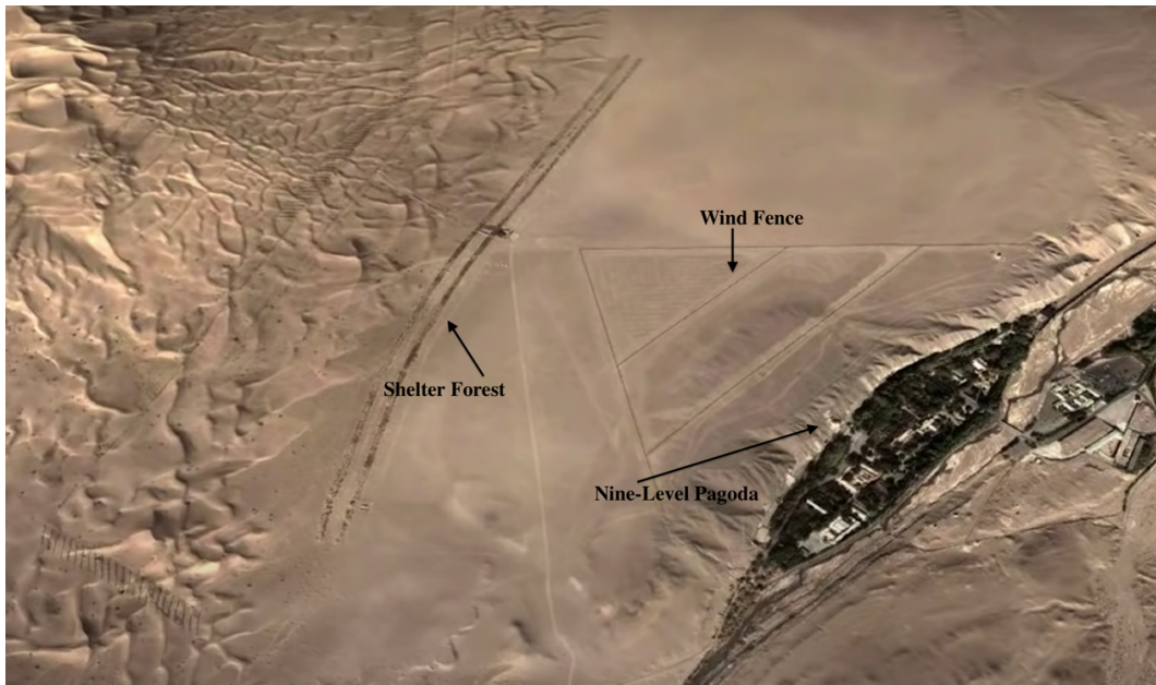
Figure 3.14: Sand control project at Mogao Grottoes. In the middle of the picture is double 2km-long anti-sand forest strips planted with sand plants such as Haloxylon and Shaguai Jujube , as well as “A”-shaped high vertical nylon anti-sand nets. Source: Google Earth
