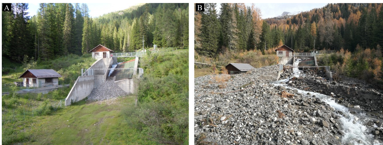
Figure 2.6 Bedload storage area (A) pre- and (B) post-October 2018 flood.
