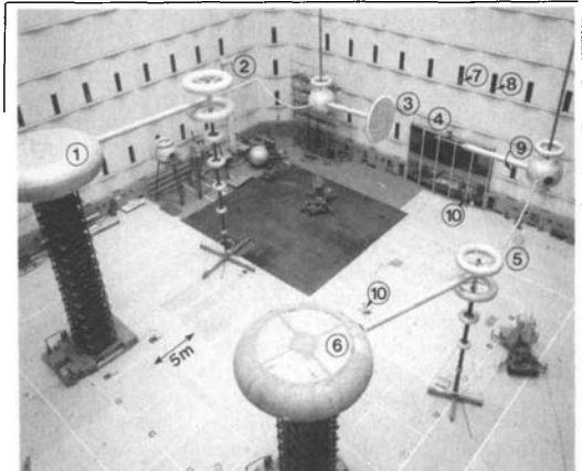
Fig. 1 View of the test circuit with conic rod-plane gap
