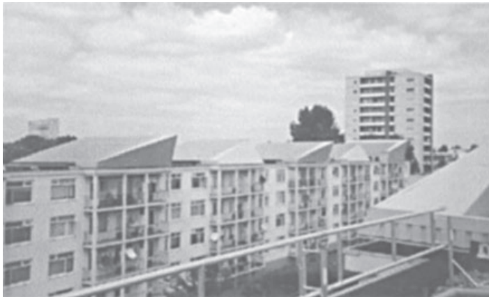
Figure 29. Solar collector modules on the roofs of the apartment blocks.
