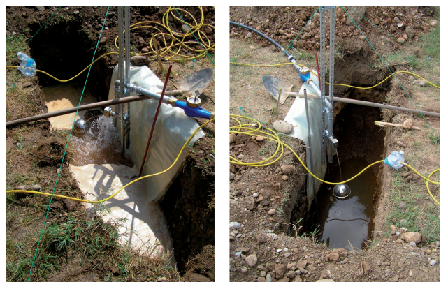
FIGURE 4 Water injection in the purpose-dug trench at the Gorgonzola site, July 2005.
