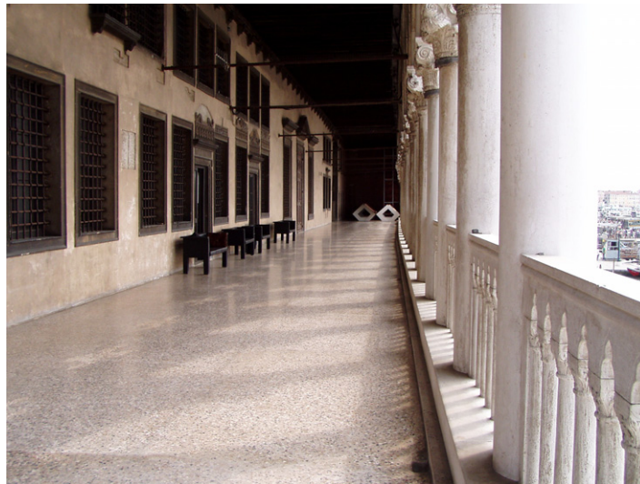
Figure A.7. Lobby of Palazzo Ducale, 50 m long: location of the receiving station.
