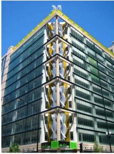
Fig. 2: Greenway Garage, Chicago (Illinois) (from: [7] [8])
