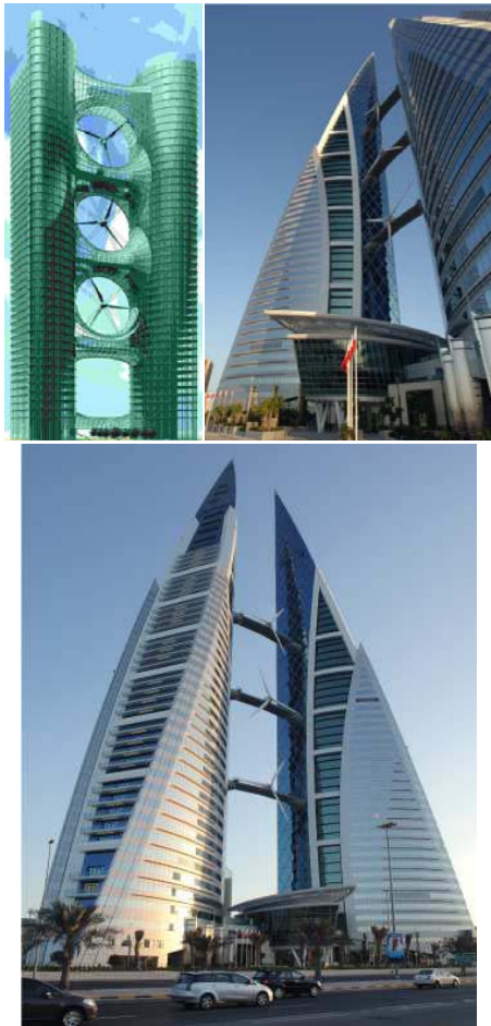
Fig. 3: a) Airfoil shaped building proposed by Campbell and Stankovich (from: [6]); b-c) WTC of Bahrain (from: [9])
