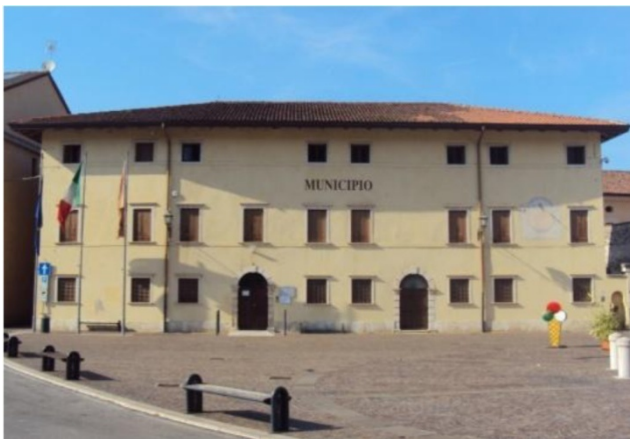
Figure 6. View of the town hall façade of Palazzo Panizza facing the triangular piazza of the town. Current condition. The recomposition of the confused space between the back of Palazzo Panizza and St. Peters church is the theme illustrated in these pages. Photo by the student Luca Costa.
