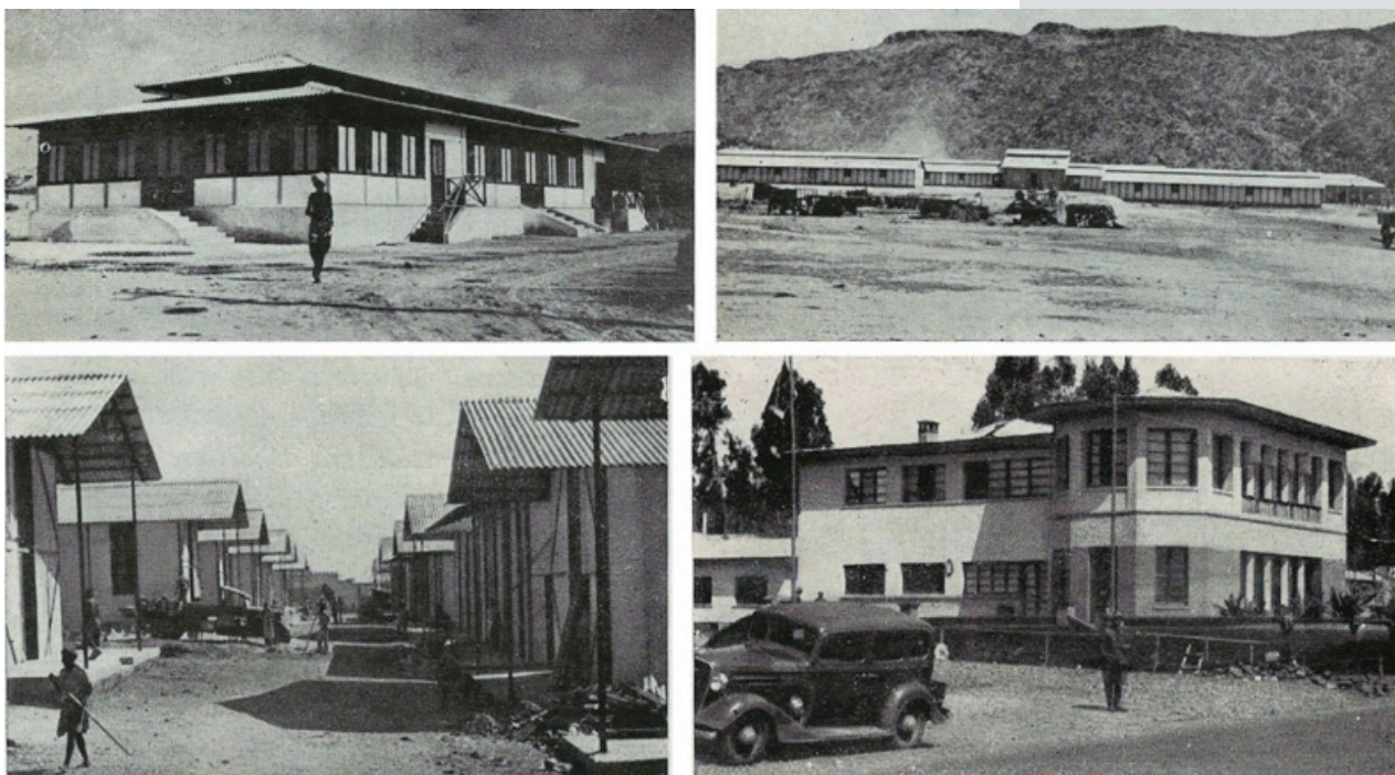
Figure 3. Buildings in East Africa that employed Eraclit panels: bungalow in Mogadiscio, camp in Decameré, Mogadiscio hospital wards and elegant house for officers in Addis Abeba. From «Eraclit», (1940), n.12, p. 12.
