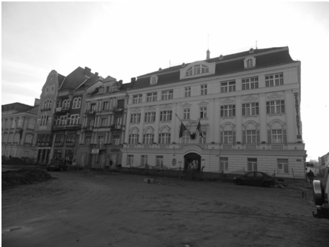
Figure 2. Buildings belonging to Timisoara historical city centre.
