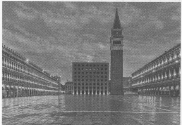
Figure 10: The metaphysical architecture of Aldo Rossi (with Gianni Braghieri) built in Modena as an ossuary that substitutes the basilica di San Marco (St. Marks Basilica) in Venice alongside palazzo Ducale. From the work of the students Enrico Palladin e Marco Ragagnin.
