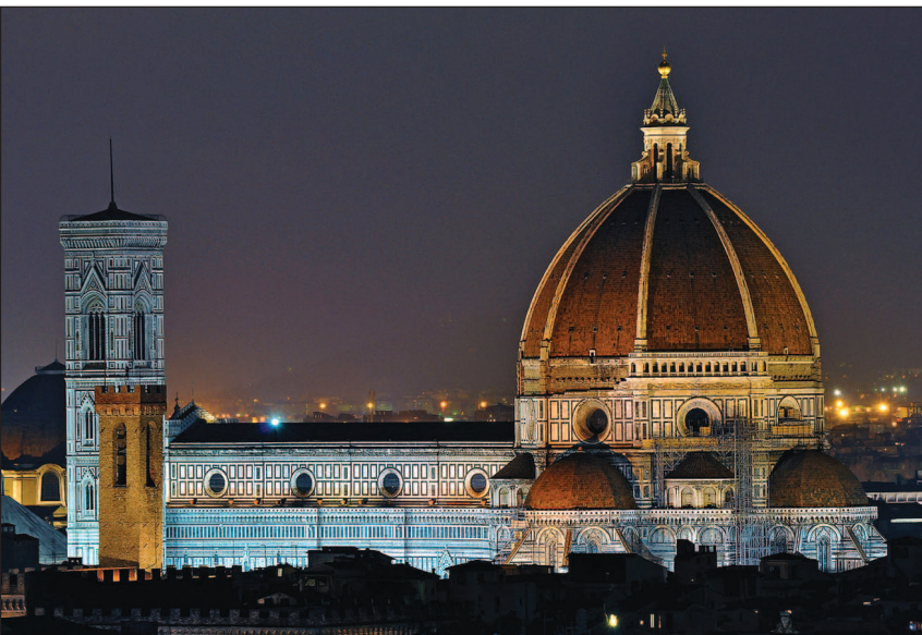
FIGURE 3 – The shortage of wood induced Filippo Brunelleschi to invent revolutionary techniques to build the magnificent and still unmatched masonry dome of the Florence Cathedral in 1420. (Courtesy of Pino Grasso.)
