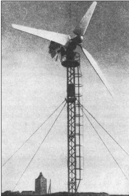
FIGURE 5 – A wind turbine installed on the tidal island of Neuwerk, Germany, in 1946. It had a 15-m rotor atop a guyed steel lattice tower with mechanical transmission to an 18-kW generator located at ground level. It was provided with automatic rotor positioning depending on the wind velocity. (Photo courtesy of IEEE Power & Energy Magazine , vol. 7, no. 5, 2009.)
