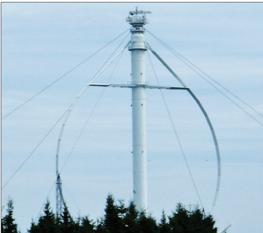
FIGURE 8 – The Éole, a 4-MW 110-m Darrieus's vertical-axis wind turbine installed at Cap Chat, Gaspésie, Quebec, in 1987 is still the largest in the world. A fault in the base bearing put it permanently out of service in 1993.
