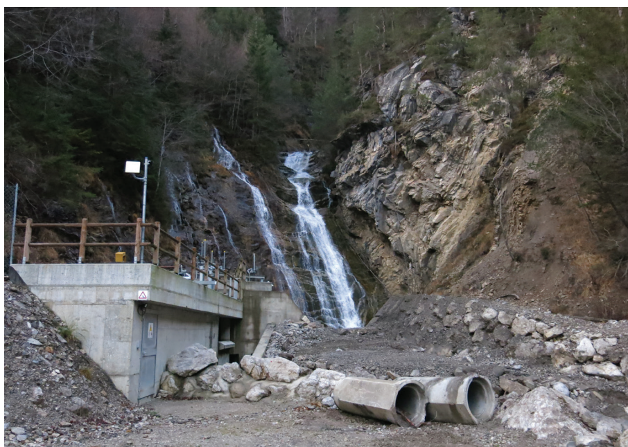
Fig. 28: Small hydropower plant on the Velezza stream in Lozzo di Cadore, Belluno province. Photograph: Giovanna Deppi
