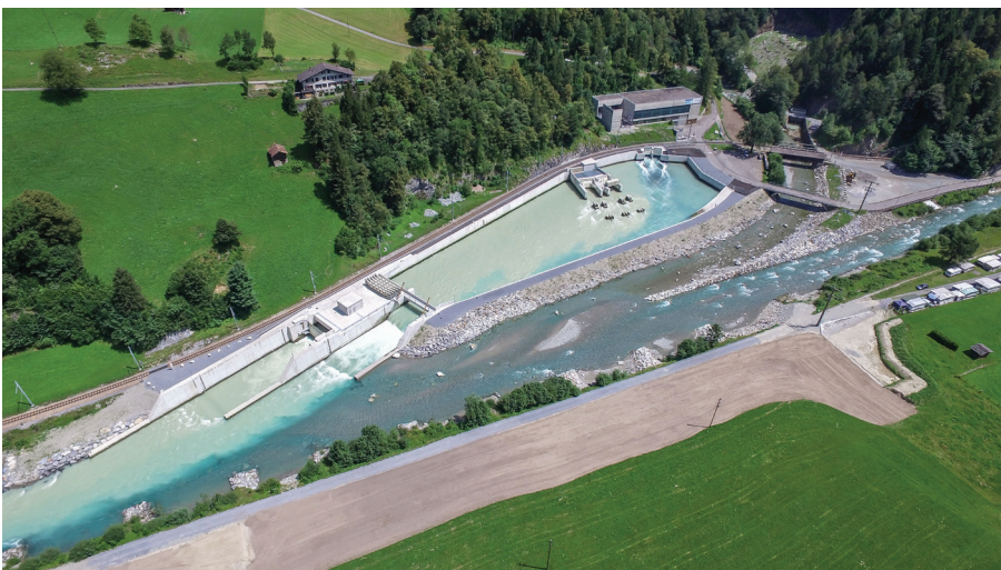
Fig. 10: Hydro-peaking stilling basin at Innertkirchen, Switzerland (Photograph © Kraftwerke Oberhasli AG)
