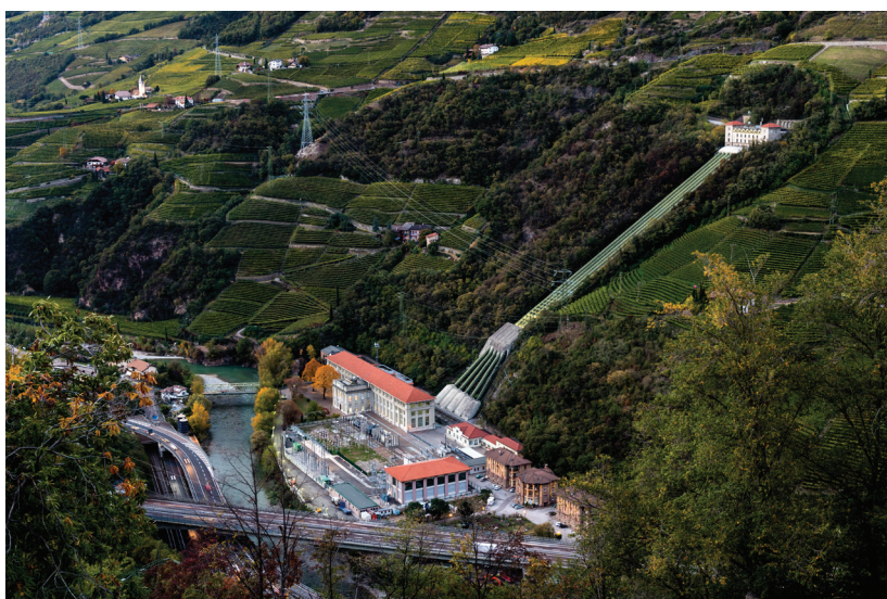
Fig. 26: Hydropower plant Kardaun, South Tyrol. Photograph: Alperia
