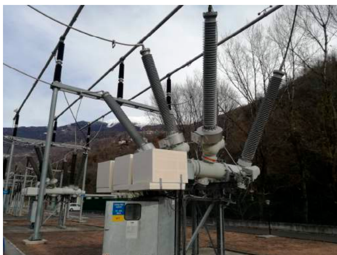
Figure 17. TSG with drives shielded by polystyrene enclosures.
