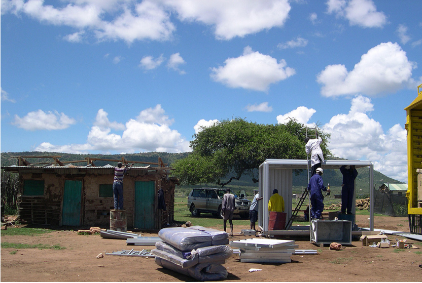
Figure 36: On-site construction of a Solarkiosk.
