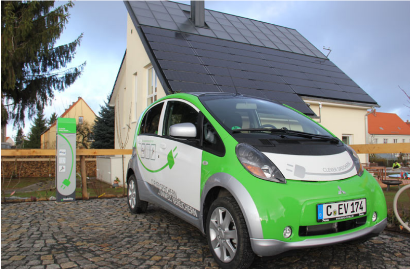
Figure 24: Energy-autonomous, single-family house in Freiberg.
