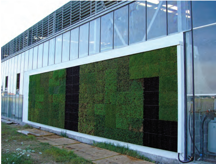
FIGURE 11. Wall installation with vertical turf with its irrigation and fertilization system integrated into the façade system.
