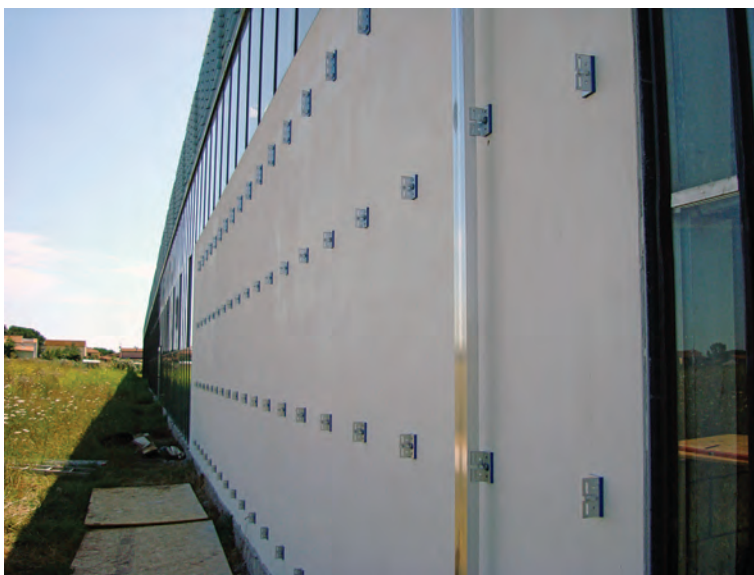
FIGURE 8. Detail of the fixing points of the panels.
