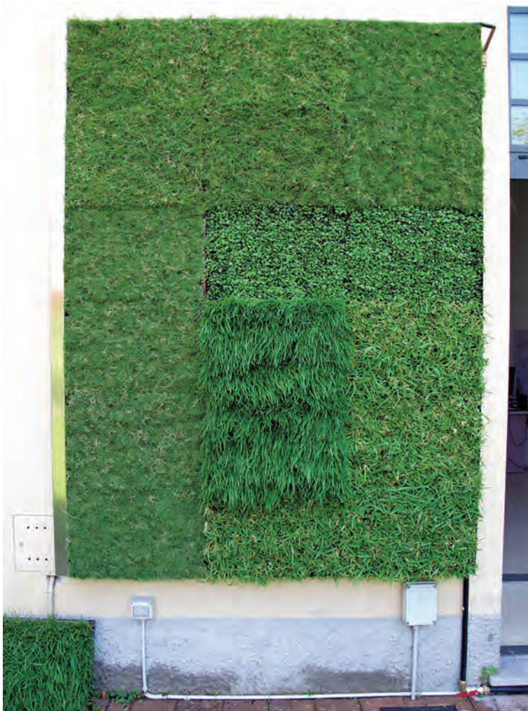
FIGURE 4. Installation of vertical turf with different species of grass.
