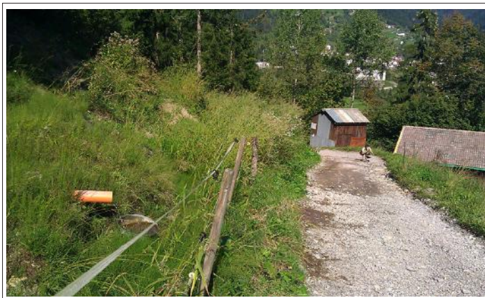
Figure 3 - Case study P1 of Paularo showing a section of a forest road where there is a clear evidence of water flow interception. In the figure also a simple drainage system is shown.
