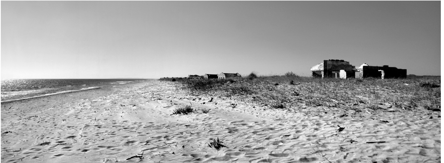
Fig. 6. Spiantza, Pyrgos Ilias, GR; abandoned houses along Anemochori coastal segment (photo credits: S. Antoniadis, 2019).
